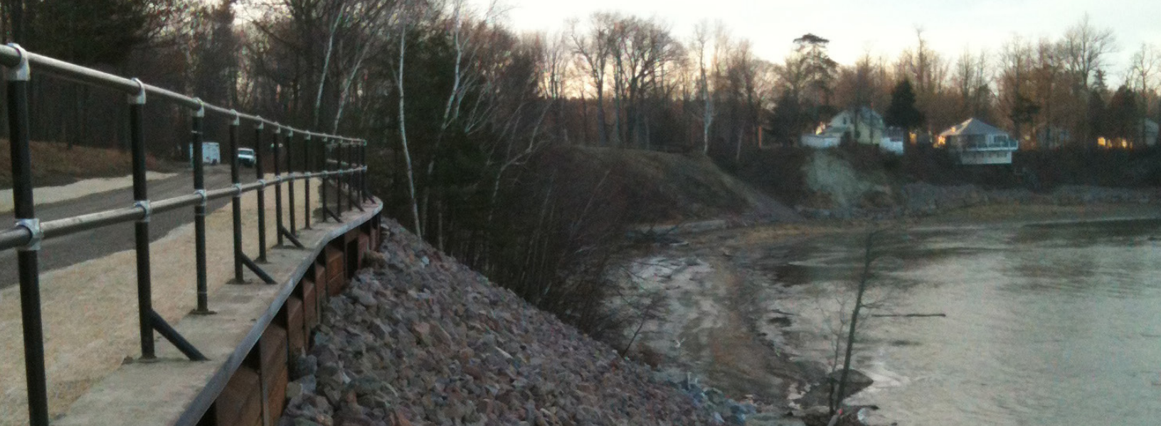
Burlington Bike Path Slope Repair, Burlington, Vermont
